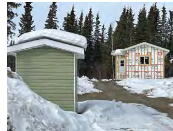
LSCFN house in progress
