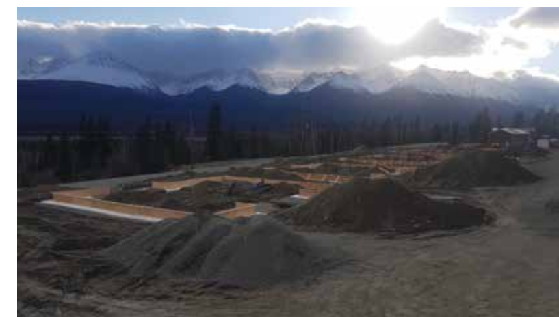
CAFN house footings, with the St. Elias Range as backdrop
