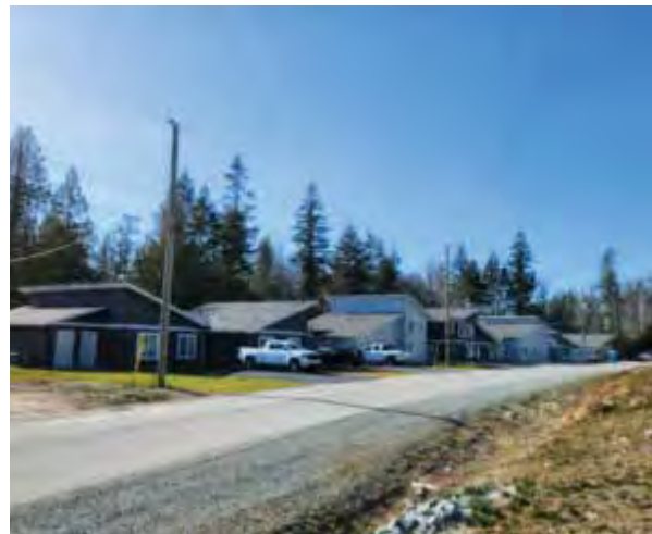
Tla'amin Nation housing multiplex under construction in early 2022, and completed homes, March 2023
