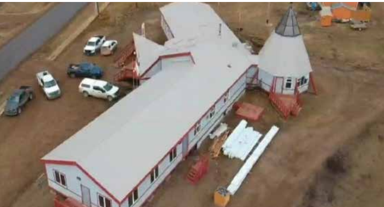
John Tetso Building construction
