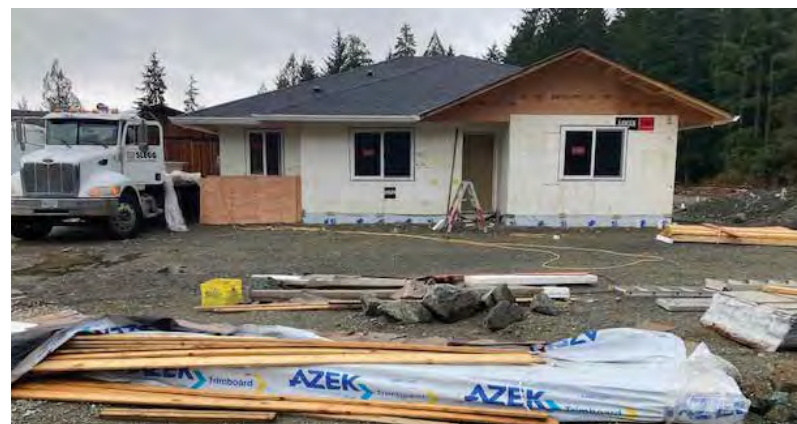
Toquaht Nation homes in progress
