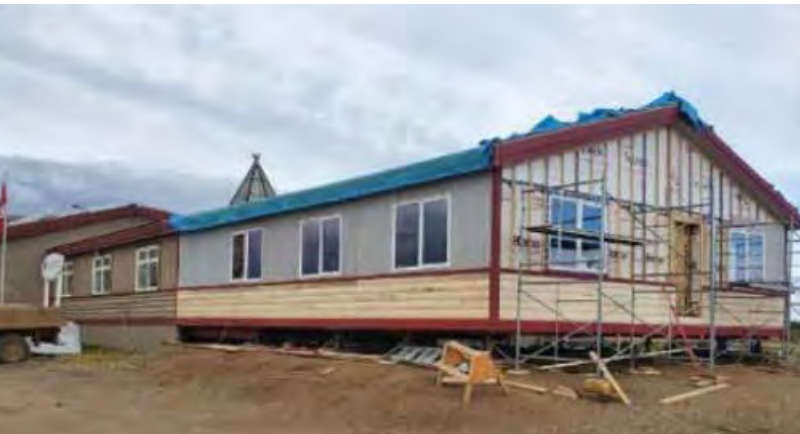
Déłıne John Tetso Building addition in progress
