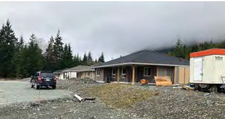
Toquaht Nation homes in progress
