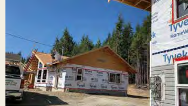
Huu-ay-aht First Nations house construction
